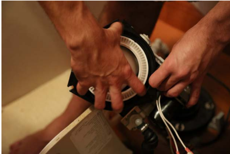
Place flush ball ring back into position (the white ring in photo)
