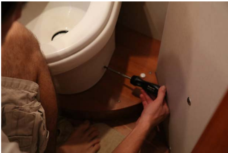
Loosen the two screws holding head to base
