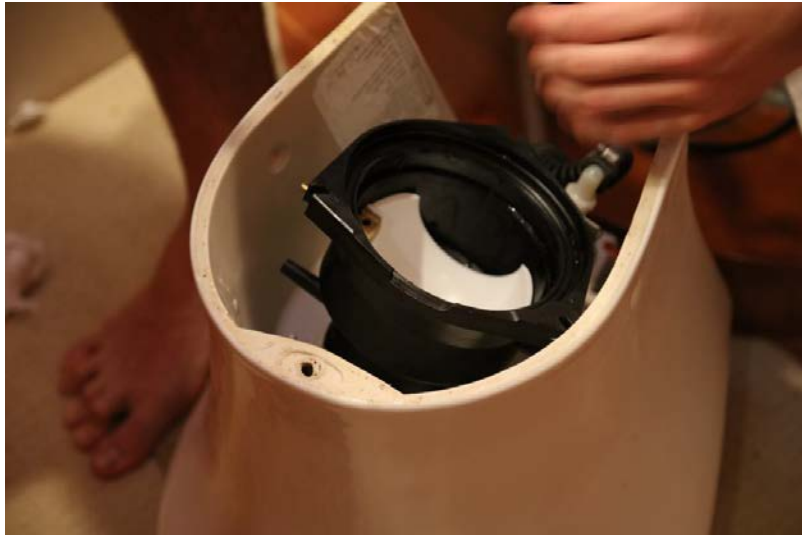
Place new shaft in hole and replace flush ball
