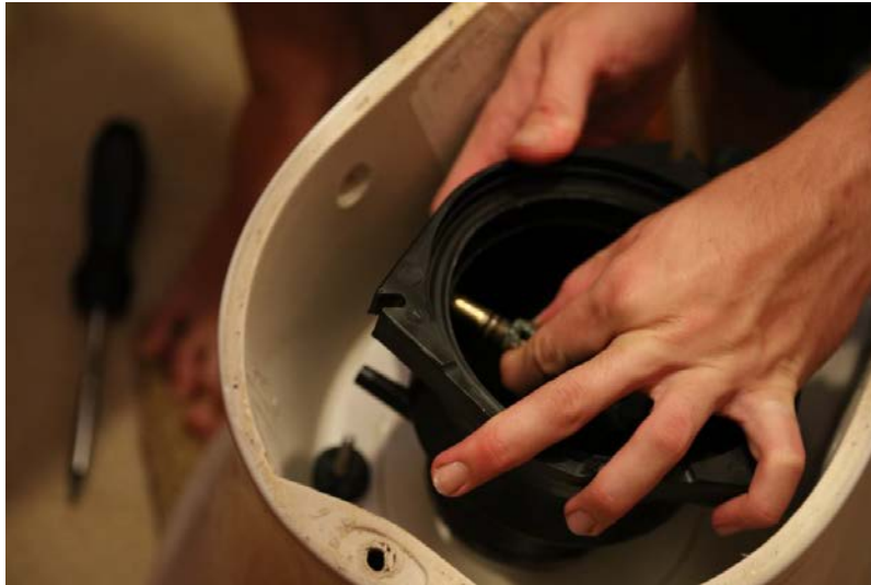
Remove old flush ball shaft
