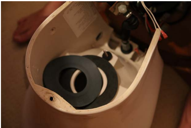
Place new seals into position – note make sure top seal is the right side up as marked
