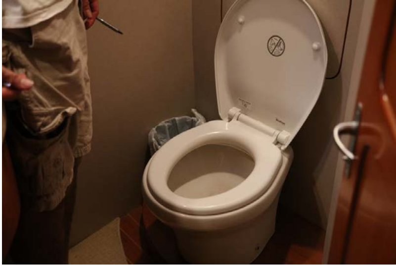
The job begins!
