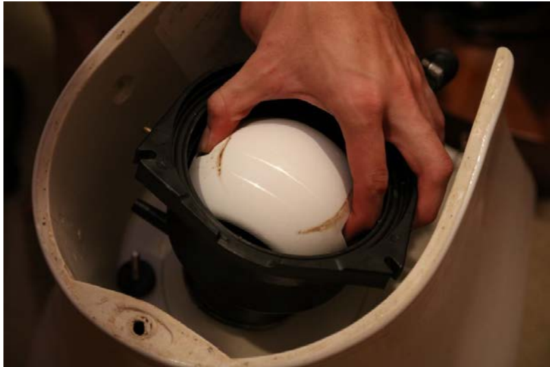
Rotate flush ball back to remove
