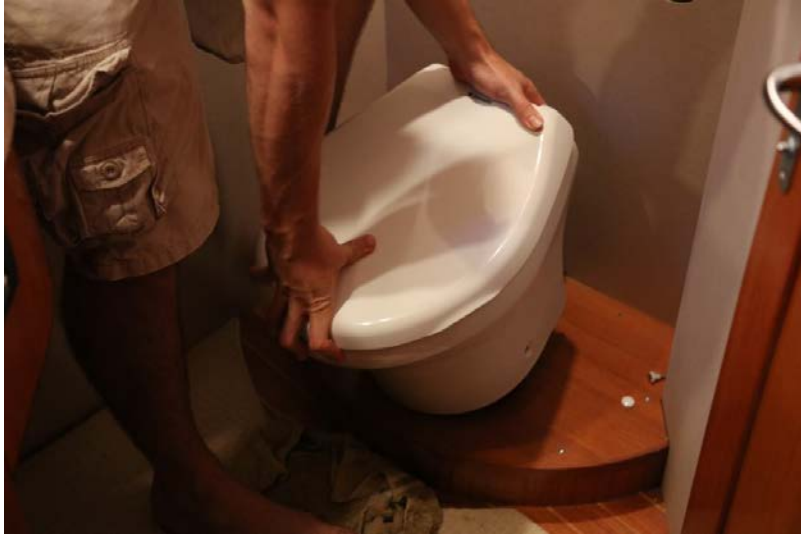
Carefully lift head off mounts
