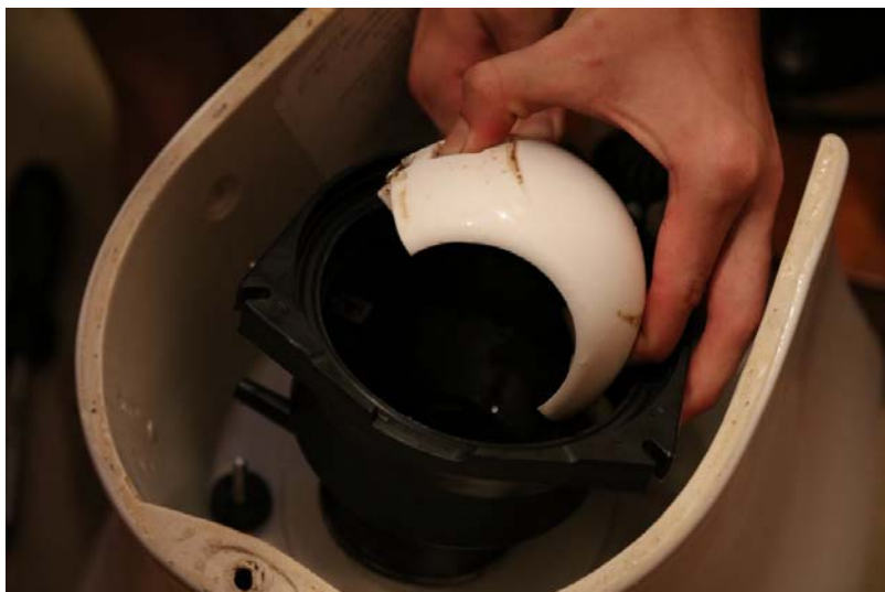
With slight pressure (pinch) remove flush ball
