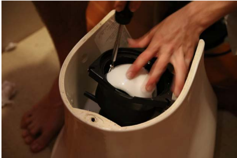
Tighten locking screw
